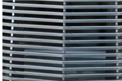
Stainless steel light mast after treatment with Steel Brite cleaning systems
