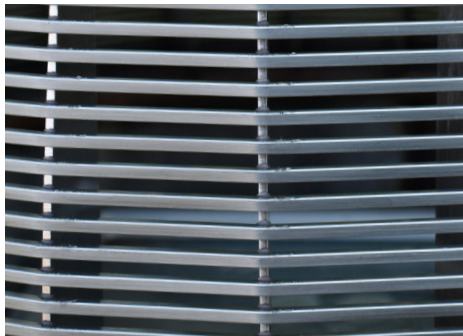
Stainless steel light mast after treatment with Steel Brite cleaning systems
